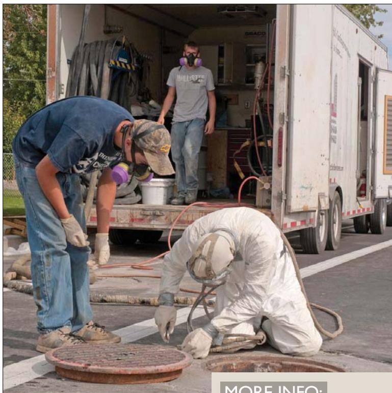
**Cody Aberasturi (in white) applies SprayWall structural polyurethane coating from Sprayroq to a manhole, assisted by Anthony Johnson and Patrick Swenson.**
